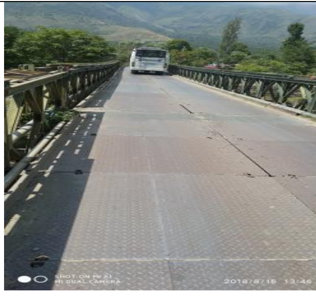
Existing Single Lane Bailey bridge on RHS of the proposed Wayil Bridge
