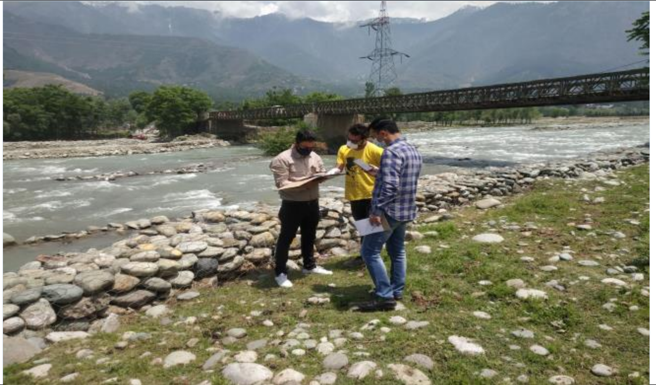
Proposed Site for Wayil Bridge
