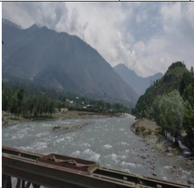
Upstream of the proposed Wayil Bridge
