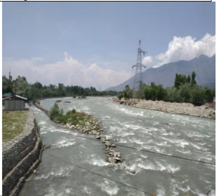
Downstream of the Proposed Wayil Bridge
